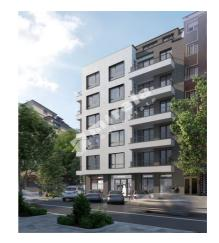
Location: Lyuben Karavelov St Construction type: reinforced concrete structure with hanging facade and brickwork Joinery: PVC five-chamber casement windows
